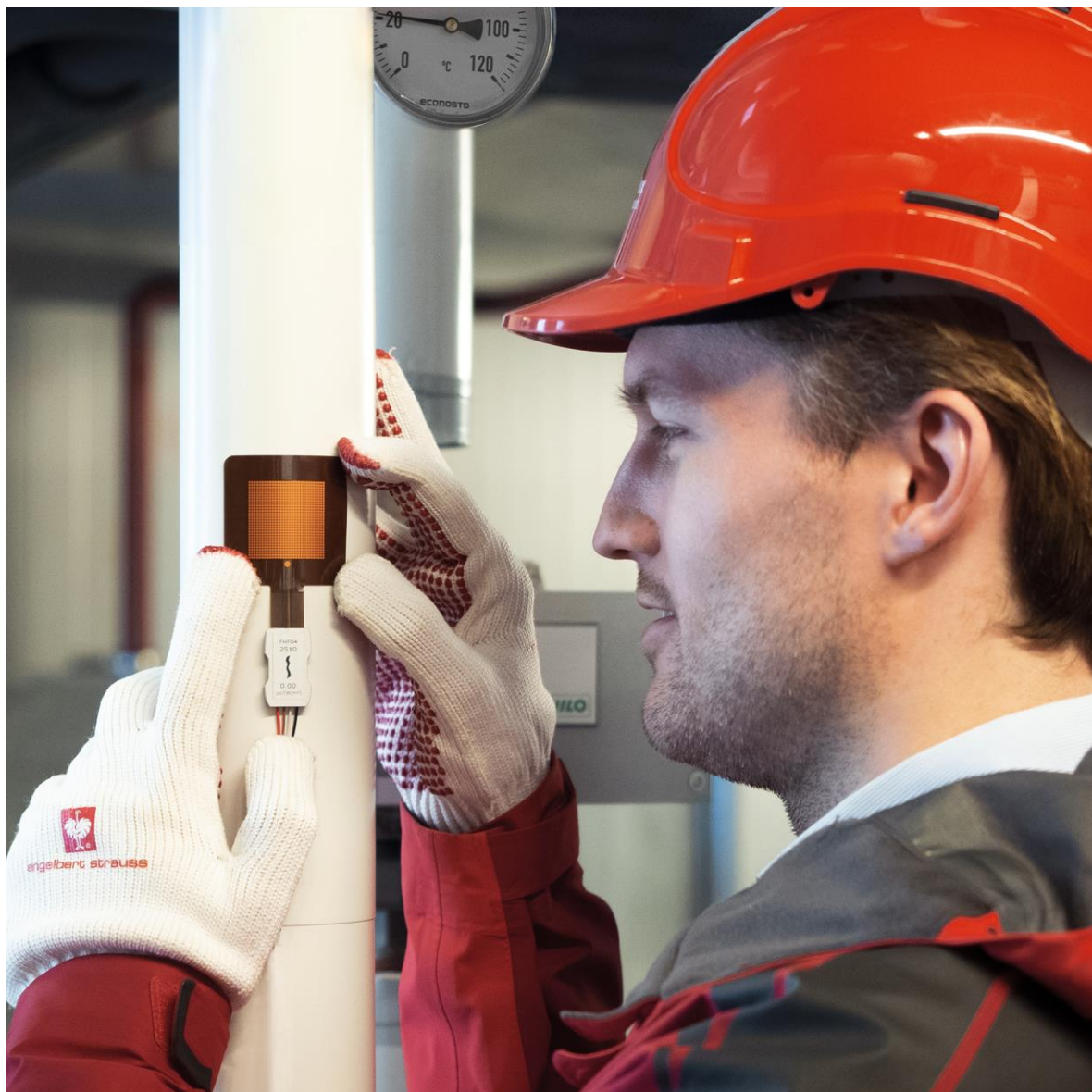
Figure 4.1.1 Example of an FHF04SC foil heat flux sensor being installed for measurement on an industrial pipe. The sensor is mounted on a well-prepared curved surface.
