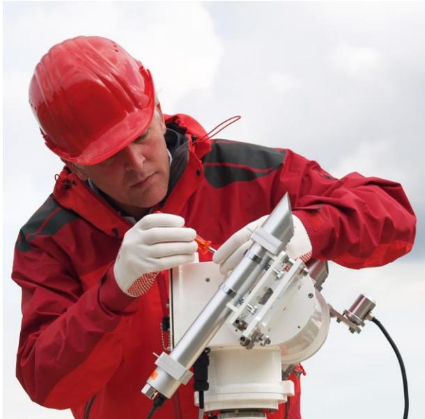
**Figure 1** installing a DR01 first class pyrheliometer
